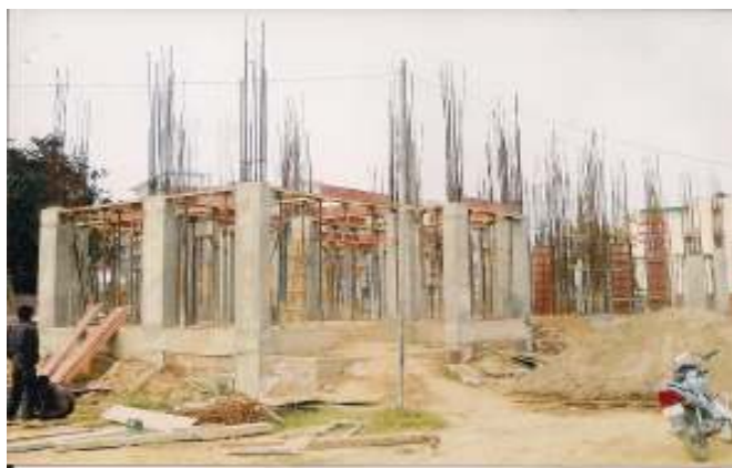
Work in progress at Zirakpur
