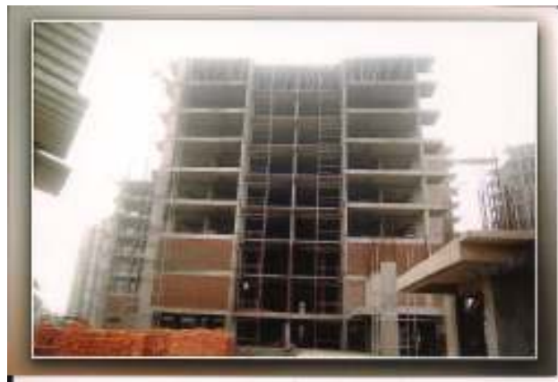
Work in progress at Sonepat
