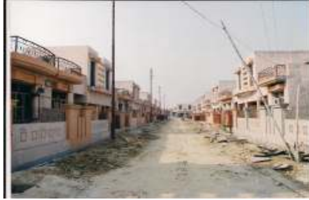
Work in progress at Lucknow Phase-III.
