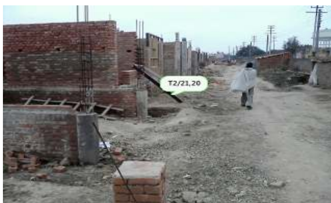
Work in progress at Meerut
