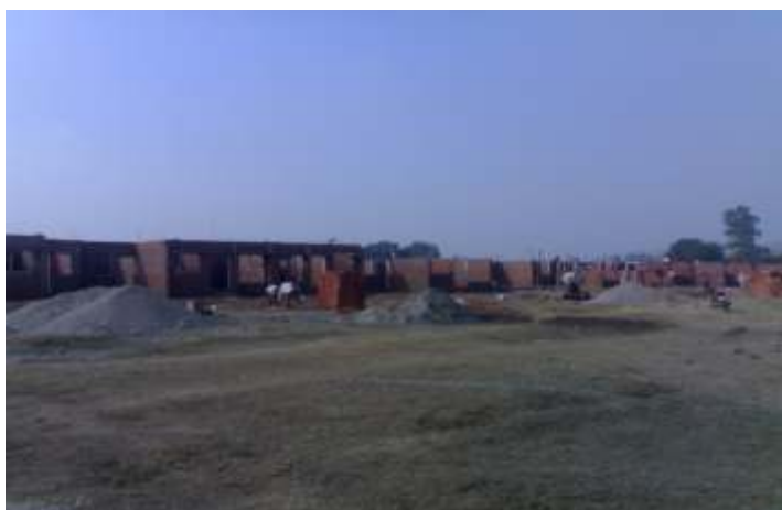
Work in progress at Moradabad
