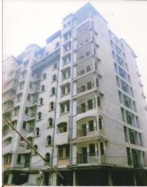
Work in progress at Kolkata Phase-III B
