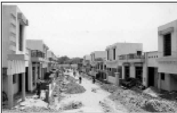
Work in progress at Lucknow Phase-III
