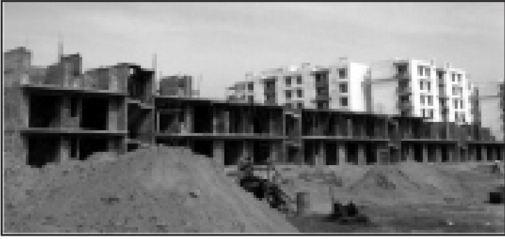
Work in progress at Zirakpur
