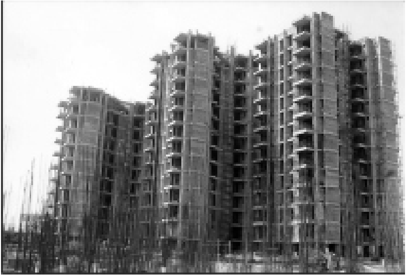
Work in progress at Sonapat.
