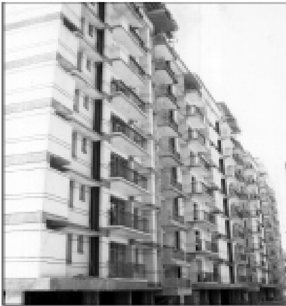
Work in progress at Vasundhara Phase-II
